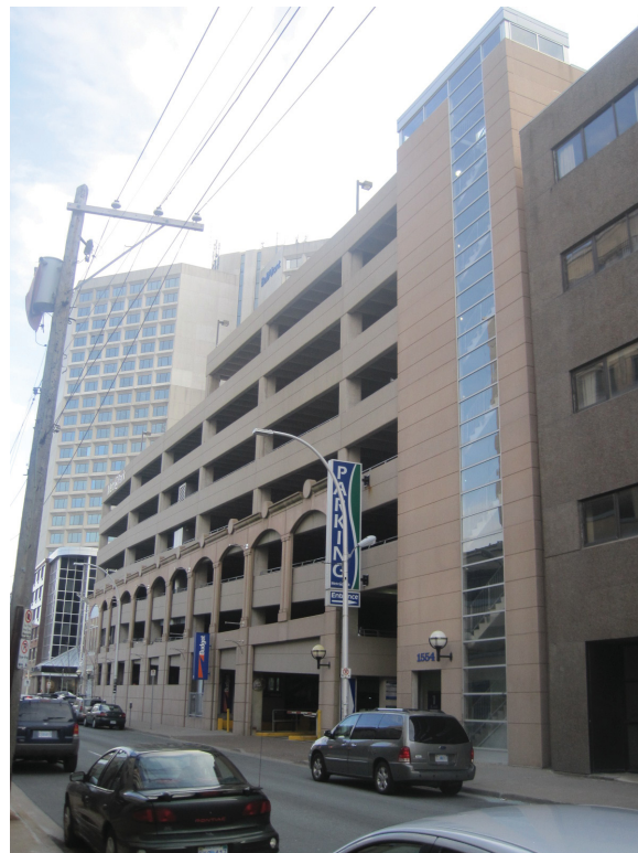
Figure 52. Hollis St. facade.
