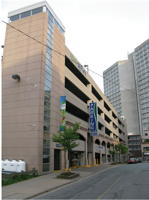
Figure 51. Granville St. facade.
