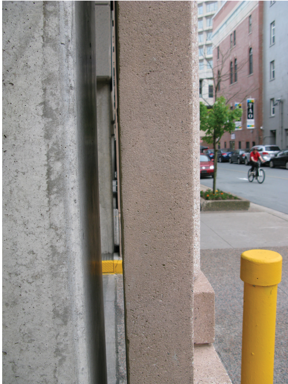
Figure 57. Detail of an existing arcade element, bolted proud of the structure.
