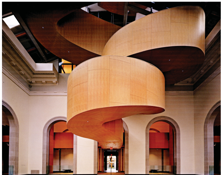
Fig.45. Spiral Staircase at the AGO. Photograph by Edward Burtynsky
