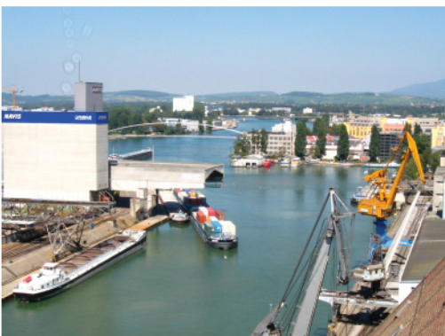
The existing Kleinmünchen port and its structures, Basel (2009).
