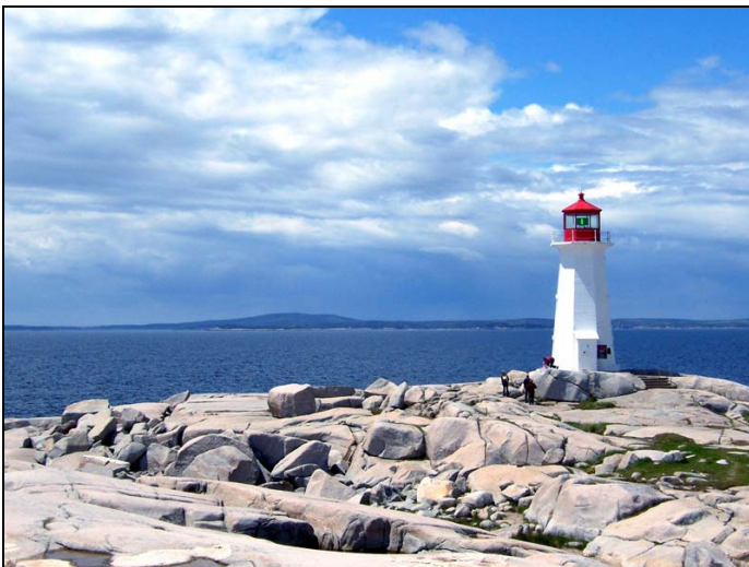
Figure 3. In addition to being a working waterfront, the fishing village and lighthouse at Peggy's Cove make it a popular tourist destination, attracting thousands of visitors each year. Source: St. Margaret's Bay Regional Tourism Development Association
