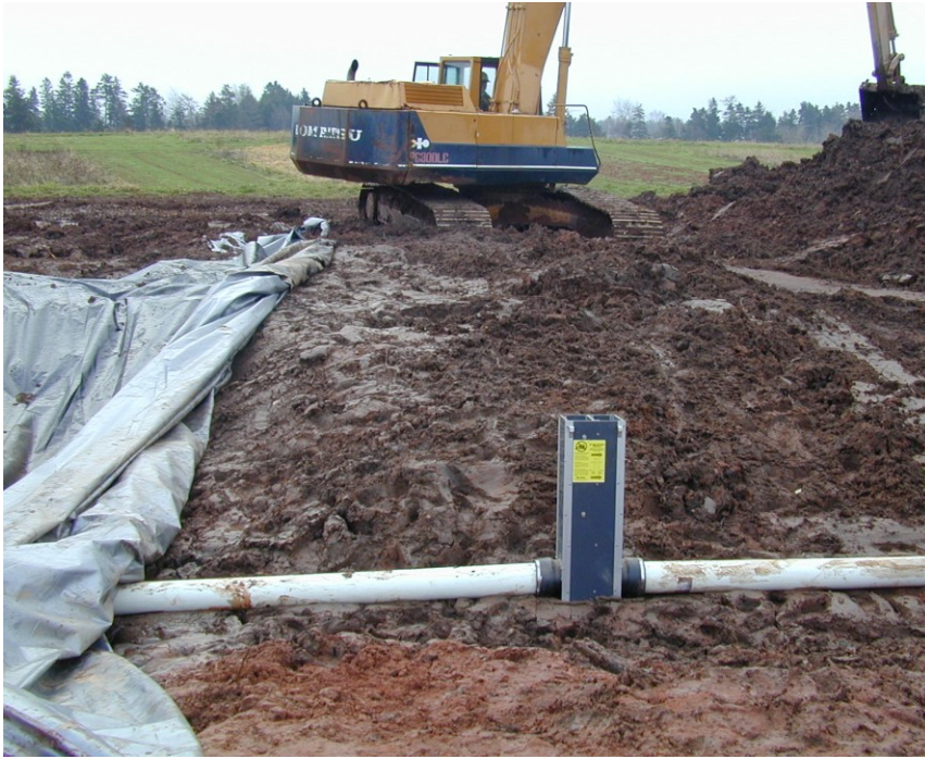
Figure 3.4 In-line control structure installation at the outlet of Wetland 2.
