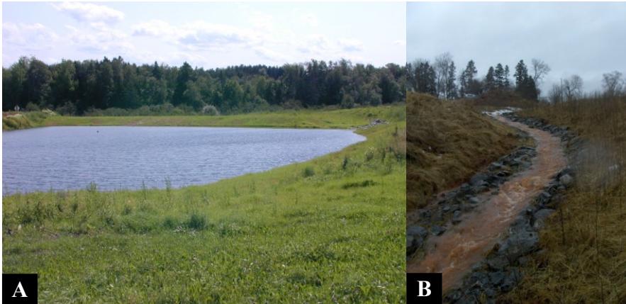
Figure 3.8 (A) Reservoir and (B) spillway.
