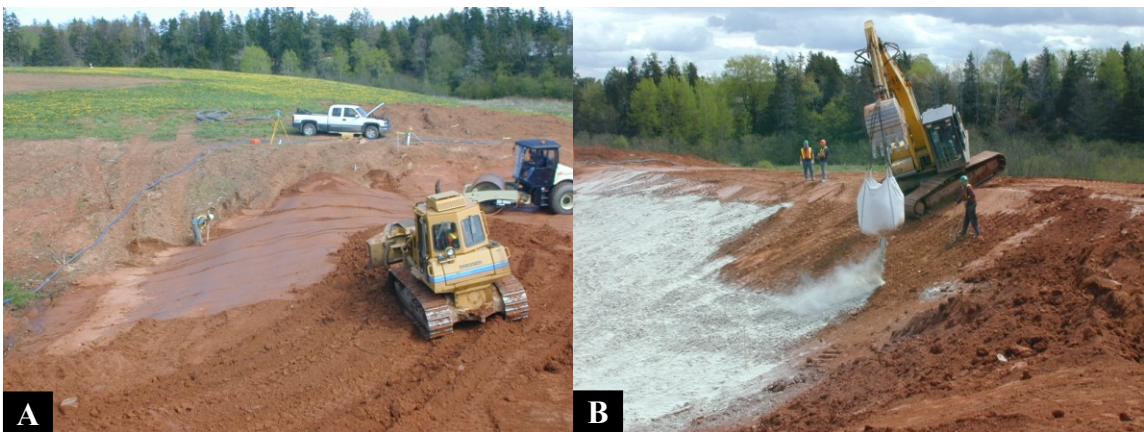
Figure 3.7 (A) Dam construction and (B) bentonite application.
