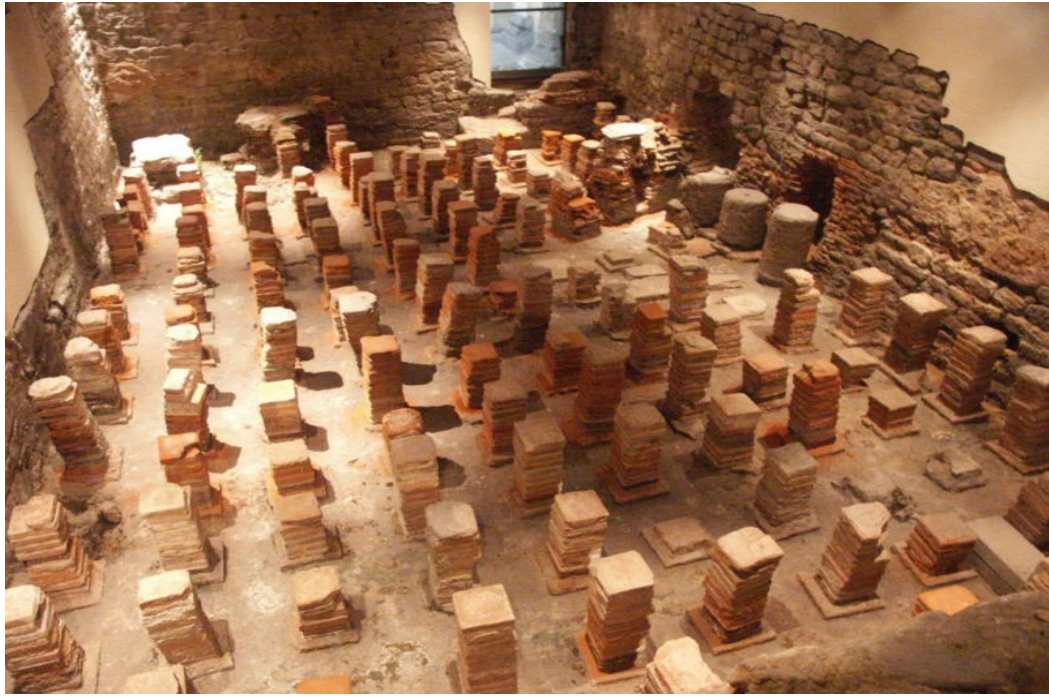
Figure 2.3: Hypocaust - under floor heating system by Romans (19) .
