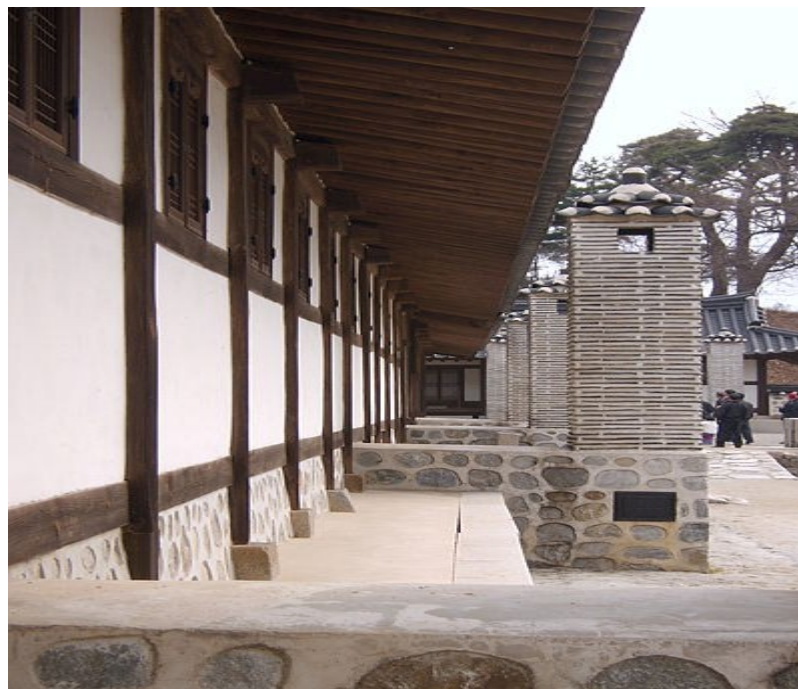
Figure 2.4: Typical high exhaust chimney in Ondol (21) system.
