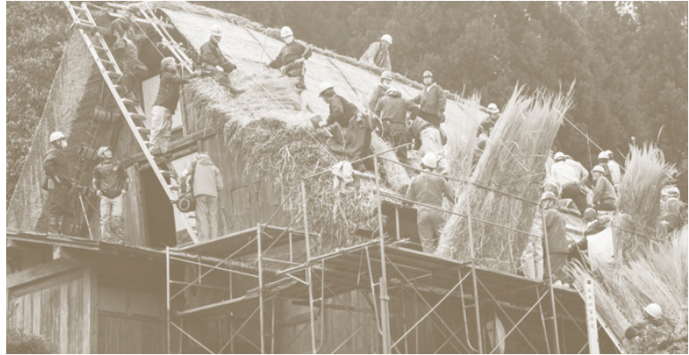
Community roof thatching (UNESCO World Heritage, n.d.).
