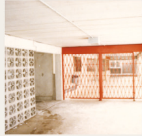
covered walkway internal gates
