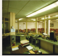
visitation control room
