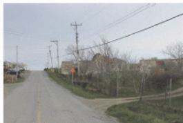
The Approach Quigley's Line
