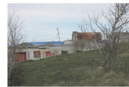
Grade Change and Crumbling
