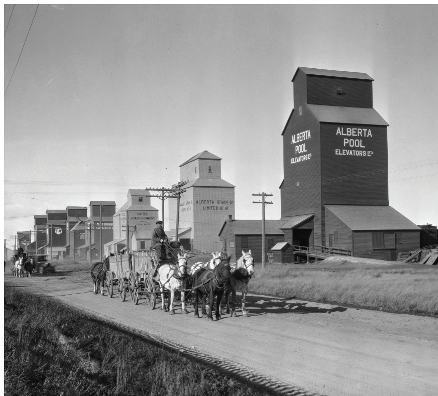
A series of elevators along the railroad tracks in Vulcan, Alberta (Oliver 1928).
