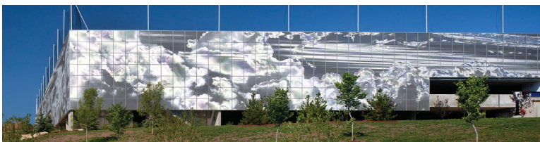
BTA's perforated cladding of the SAIT Parkade (Dan, 2011).
