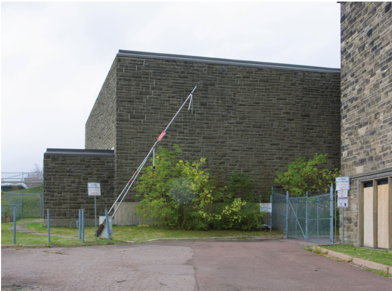
Existing Gymnasium addition and bottle necked entry to courtyard.
