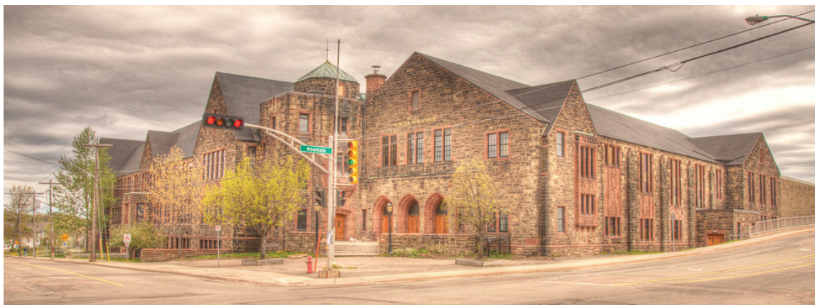
Former Moncton High School on the corner of Mountain rd. and Church st.
