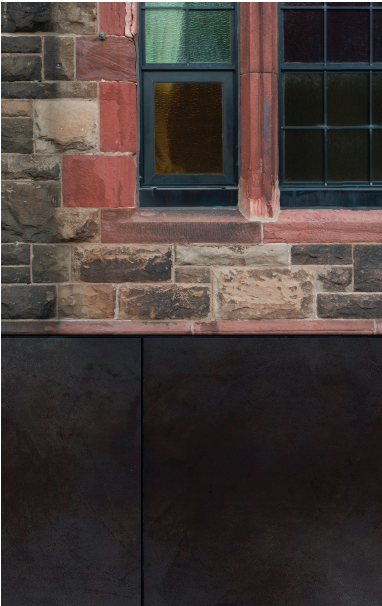
Photo collage showing introduced black oxidized steel panels and doors with existing sandstone cladding and stained glass theatre windows.
