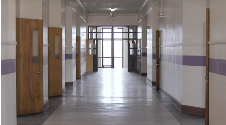
Existing state of classroom wing hallways.
