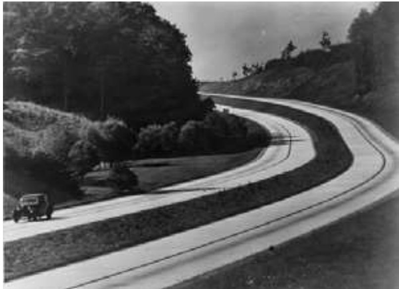
A German Autobahn in the 1930's (German-Autobahn. 2016)
