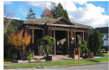
Museum at Scotia California. Neoclassical architecture adapted with materials and technology of the company town, 2010; image from Pedaling and Pedaling and Pedaling.
