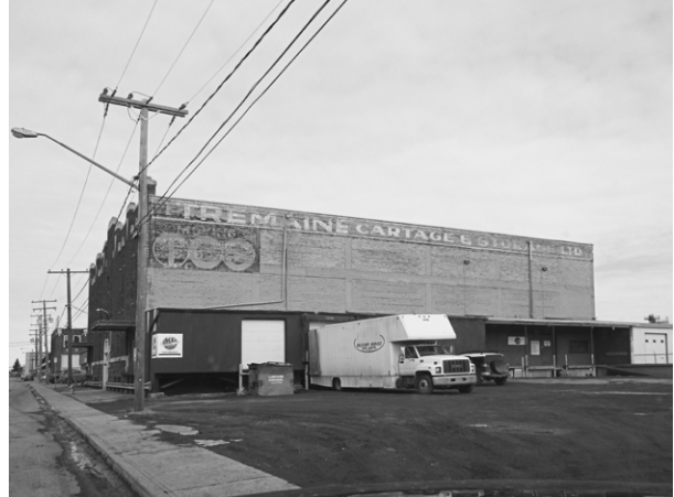
Current view the south side of the warehouse
