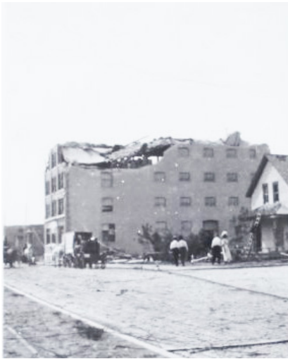
Historic image of the warehouse after the 1912 cyclone; R-A265 (1)-(29); Saskatchewan Archives
