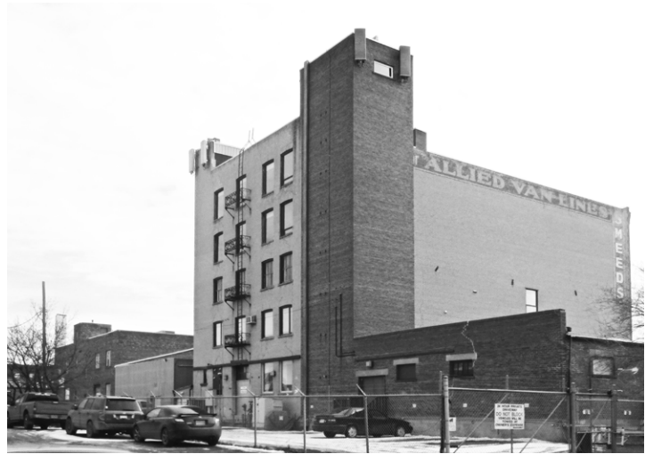
Current image of rear of the warehouse
