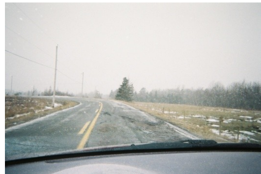
Figure 8 James' photo 2 of potholes.
