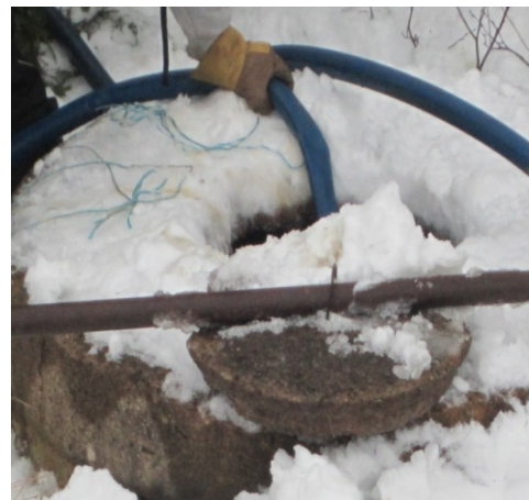
Figure 20 Martin fixing the well.
