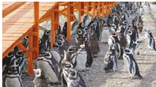
To minimize inference with the penguin population, areas of high crossing traffic are elevated to allow the penguins to walk through unimpeded
