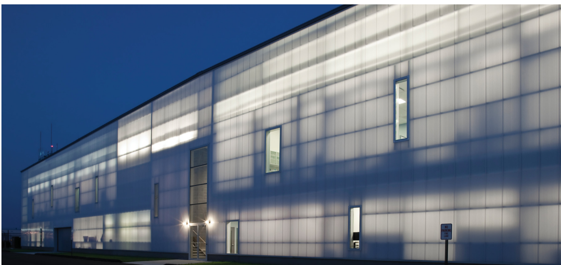
EXTECH polycarbonate translucent skin at Sikorsky Memorial Airport; from Karin, Tongue and Groove Cellular Polycarbonate Panels
