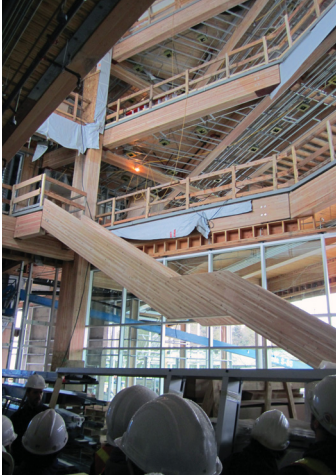
Atrium showing the use of exposed Wood Panels and Glulams
