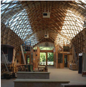
Downland Gridshell from the exterior and interior (Davey 2010)
