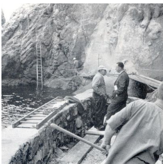
Construction of the Seawall (Vancouver Archives 1963)
