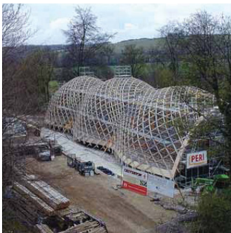
The Lowering of the Downland Gridshell (Harris 2003)
