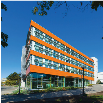
Exterior of Center for Interactive Research in Sustainability with solar aquatics located in clear view of the public in the glass viewing area on ground level (Erhardt 2011)
