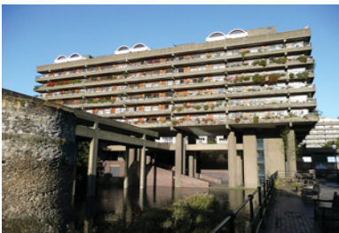
Barbican Estate Terraced block overlapping an artificial lake Photograph by EZTD
