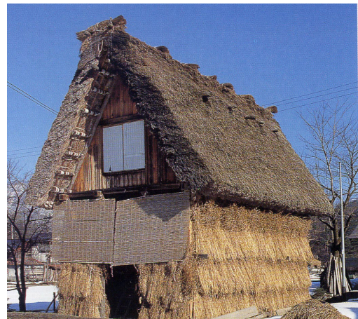
House in Shirakawa, summer condition on left, winter condition on the right. From Saito 1996.
