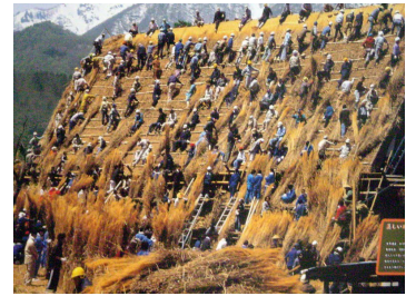
Communal thatching, Shirakawa Village. From Saito 1996.
