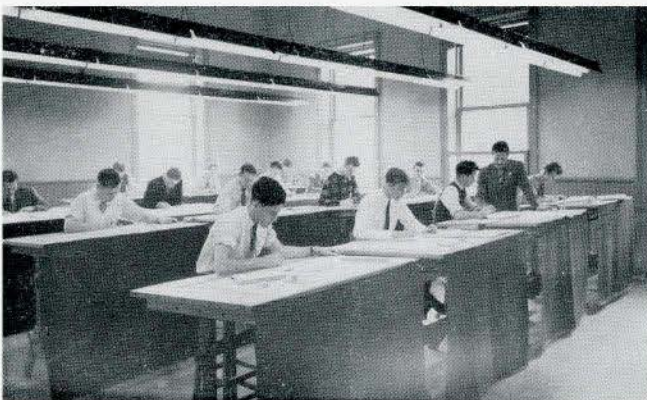
Photos courtesy of Townsend and Ibbotson
