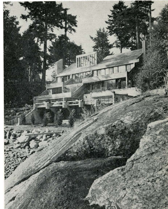
Brasso House, West Vancouver, by Anderegg and Wills. "Planning, materials and form are well used to support the grand nature of interior spaces and vista to the sea."
