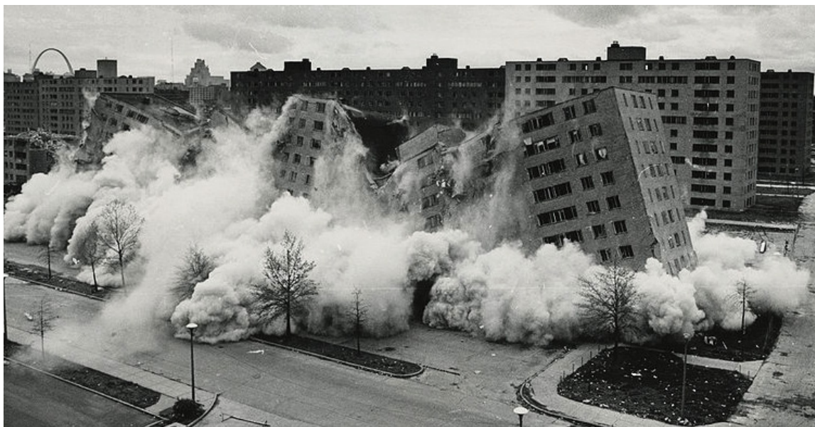
A photo showing the demolition of Pruitt Igoe in 1972 (Wikimedia, 1996)
