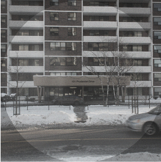
Photo of typical building type.
