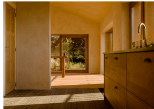
Hempcrete Interior Wall - Plaster
