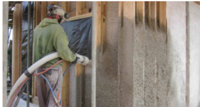
Hempcrete Wall -Spray Application
