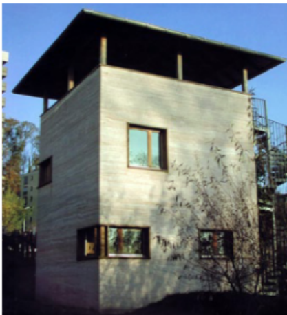
Hempcrete Exterior Wall - Plaster
