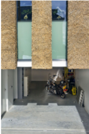
Living on the Edge. Subgrade garage entrance and straw thatch exterior finish.
