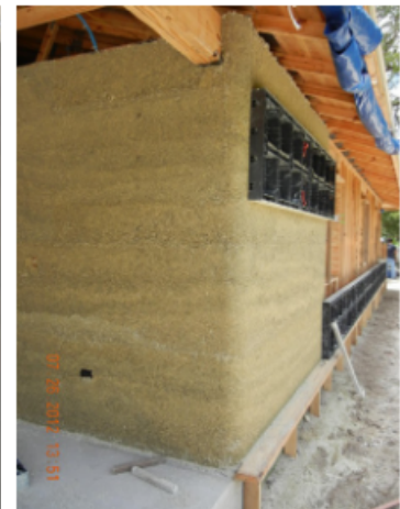
Hempcrete Wall - Cast-in-Place
