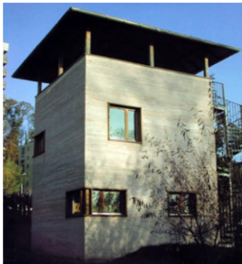
Hempcrete Exterior Wall - Plaster
