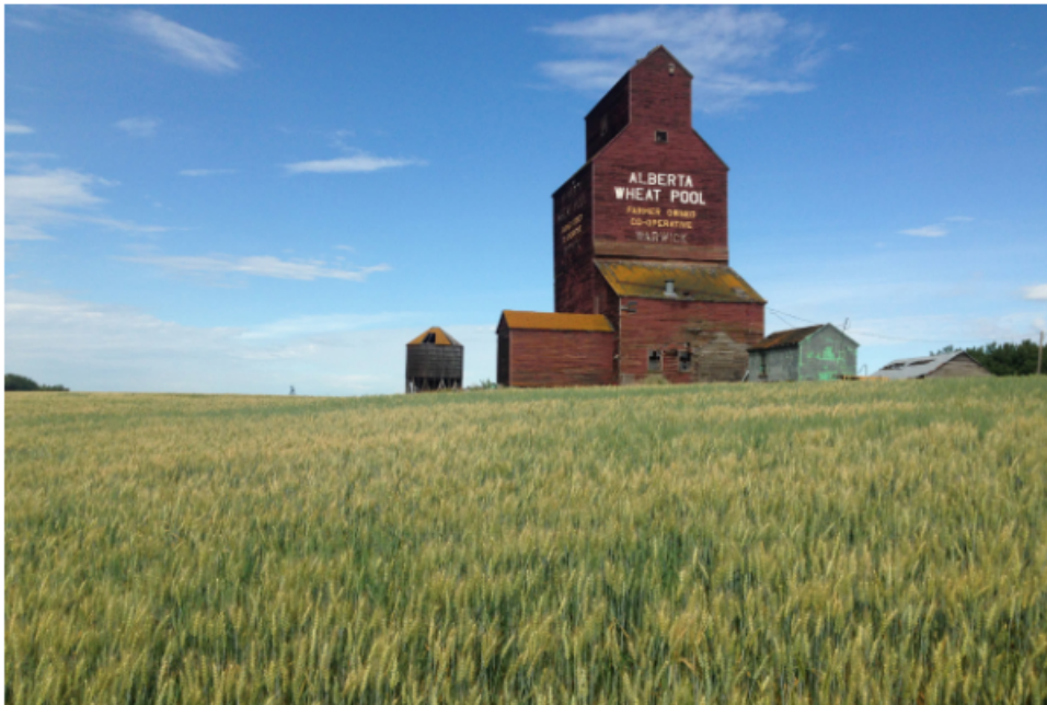
The privately operated Warwick Grain Elevator, Warwick RD, Eastern edge of Warwick Community. 2016.
