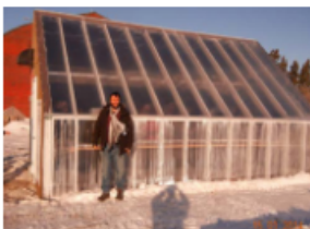
Building a Hempcrete Greenhouse. Built on organic farm operation 10 miles south of Vegreville, Alberta.
