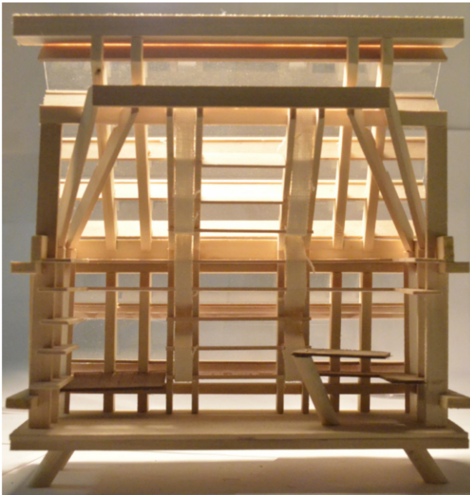
1:20 Framing Model of Greenhouse/Kitchen
