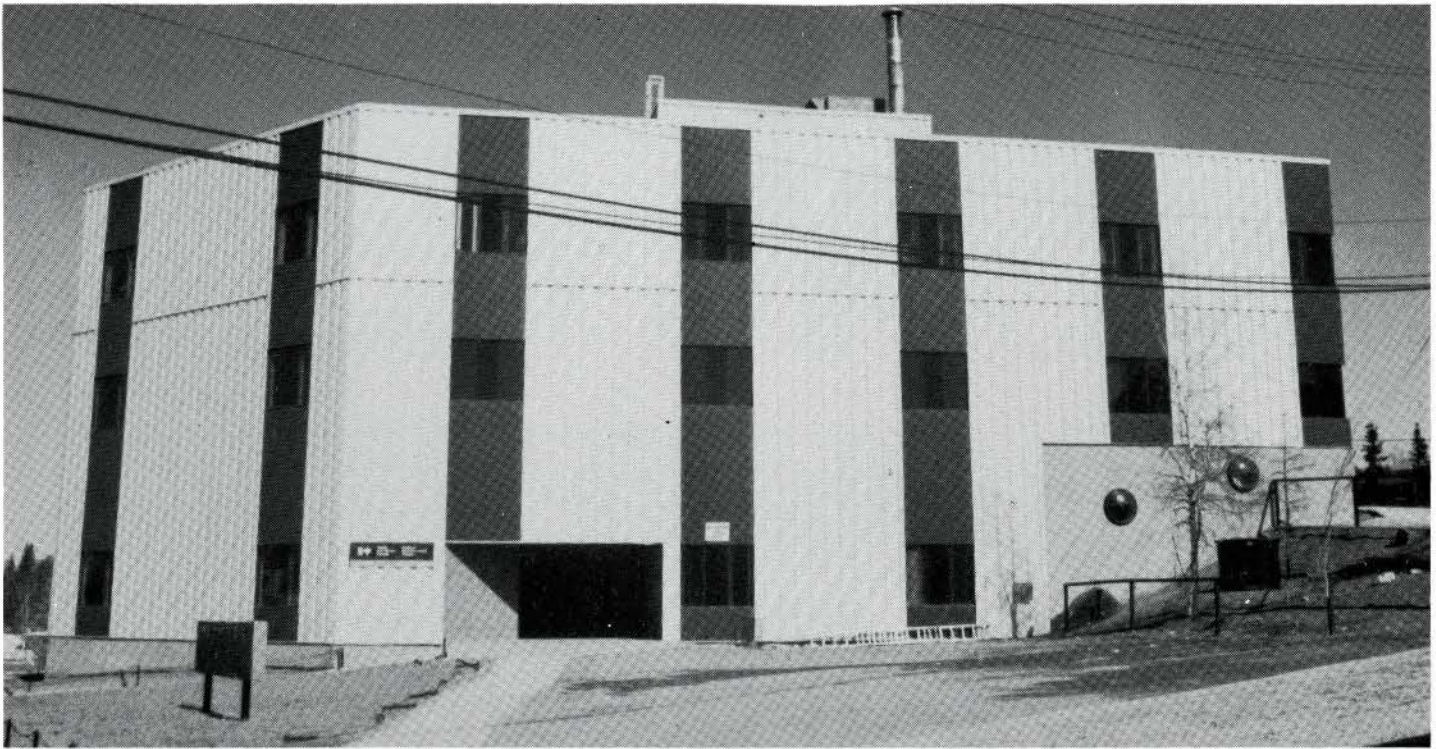
Lahm Ridge Towers a standard metal clad structure for an important city site.
