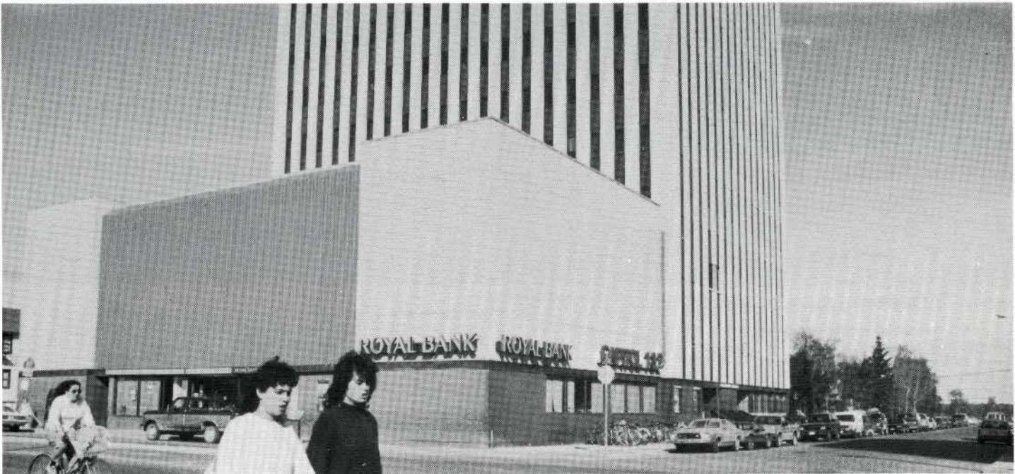
The Precambrian Building lacks the success of its predecessor, a popular movie house.
