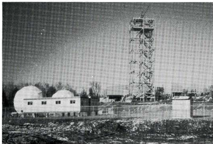
Short Range Radar Prototype under construction at North Bay, Ontario.
