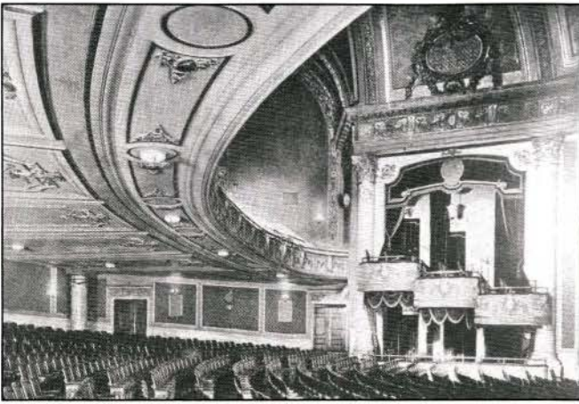
Figure 5. Lower auditorium, decorated in gilt, plaster ornament, and red brocade. (Construction)
