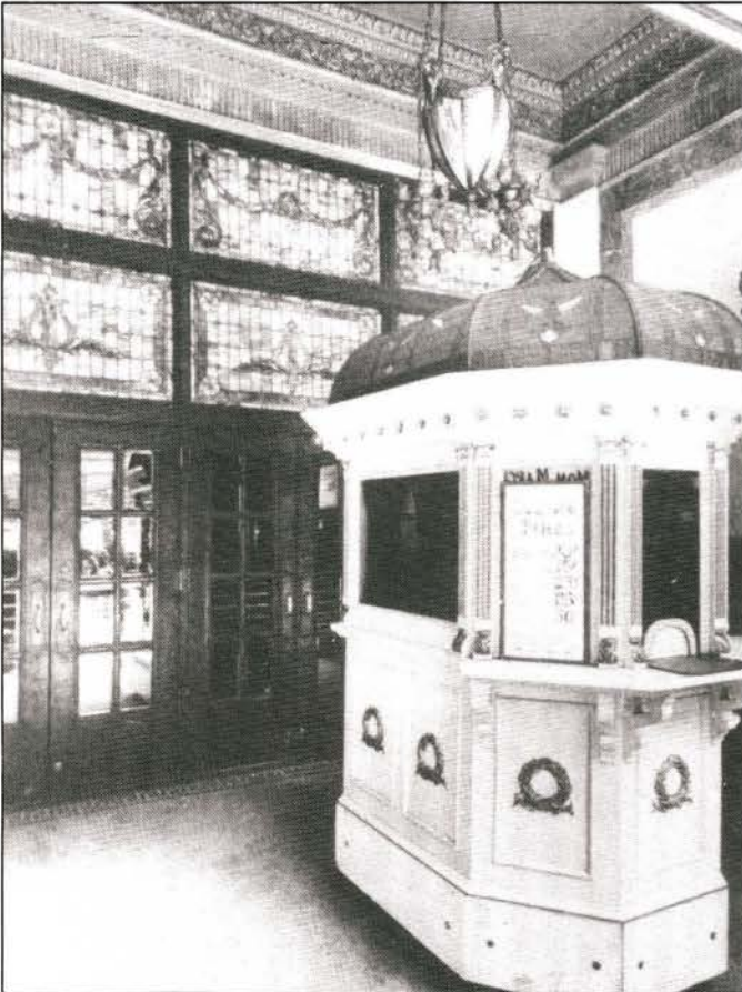
Figure 11. Exterior vestibule and ticket booth. (Construction)
