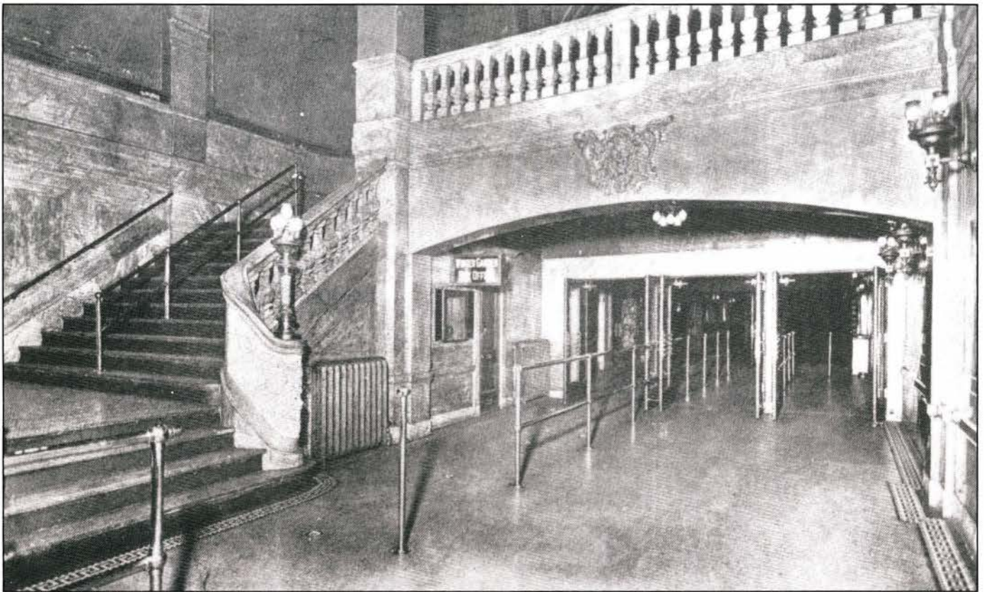
Figure 12. View of "staircase hall" and grand staircase to Winter Garden Theatre. The doorways lead to the "elevator hall," and rear entrance doors to the lower auditorium. (Construction)
