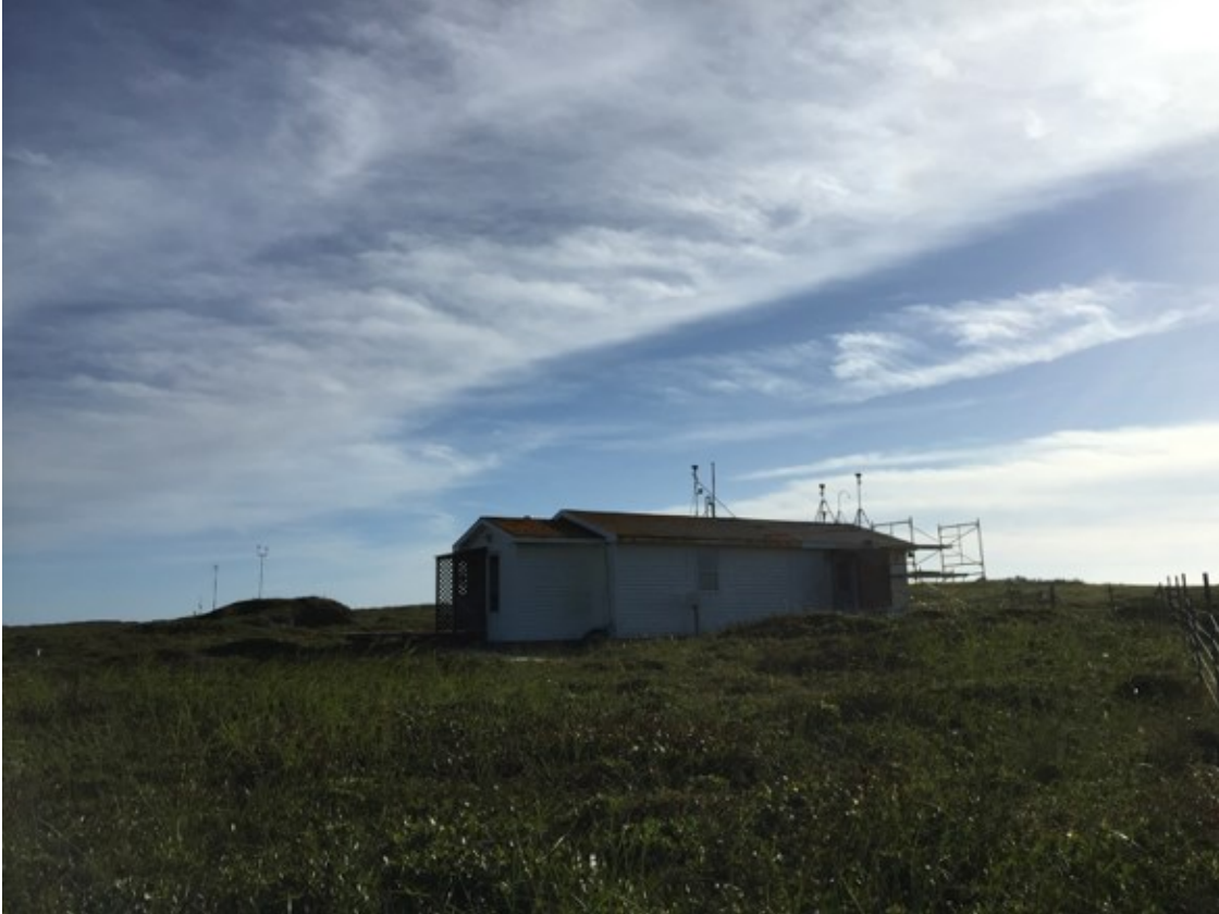
Figure 9. The Air Chemistry Monitoring Station on Sable Island
