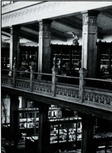
Figure 27 (above). Abstract natural motifs were incorporated into the design of the iron grillwork, the oak casework and columns, and the plaster cornices and mouldings. (Detail from a photograph in Notman Photographic Archives)
