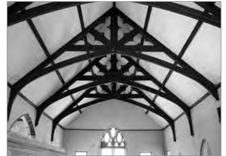
FIG. 17. PARIS TOWN HALL, ASSEMBLY ROOM ROOF. | MALCOLM THURLBY
