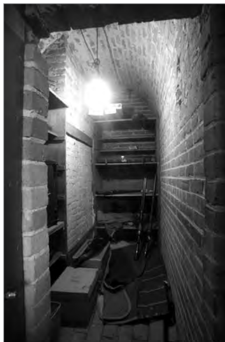
FIG. 12. PARIS TOWN HALL, GROUND FLOOR, VAULT. | MALCOLM THURLBY
