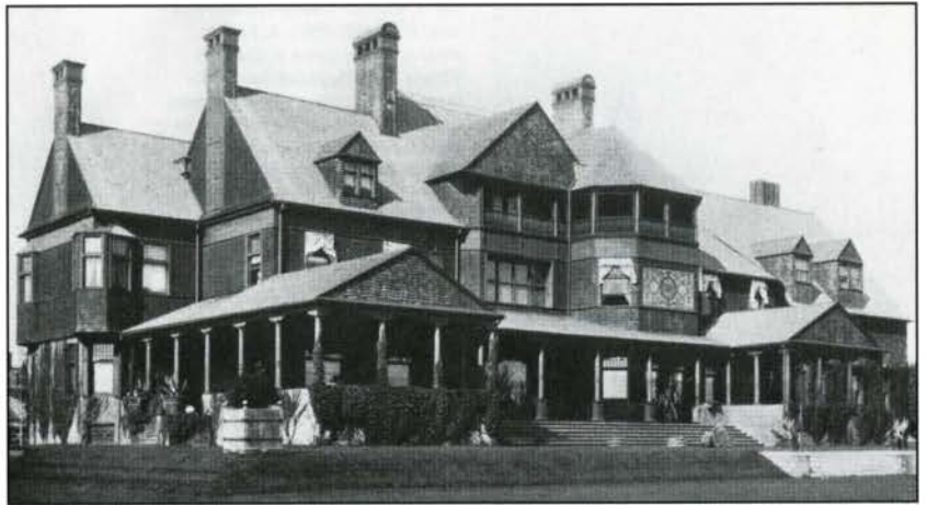
Fig. 3. "Southside", Robert Goelet's summer house in Newport Rhode Island, built between 1882 and 1884 and typical, in the grandest sense, of McKim, Mead & White's early shingle style houses with its picturesque towers, porches, dormers and chimneys all lending support to a visual delight (G.W. Sheldon, Artistic Country Seats , New York, 1886-1887, Plate 5)
