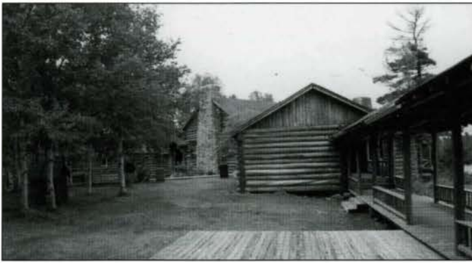
Fig. 18. The camp at Holmes Lake, northwest of Miramichi City, N.B. The main lodge is at left centre in the distance, a bedroom wing is at right centre with a covered walkway to right leading to another bedroom complex. The full log construction is evident. Summer, 1999. (New Brunswick Museum, 1999).
