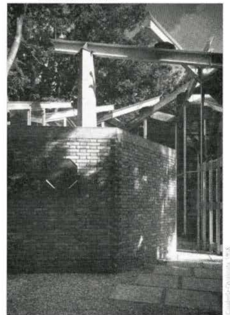
FIG. 13. VIEW OF COLUMN FROM OUTSIDE THE CANADIAN PAVILION.
