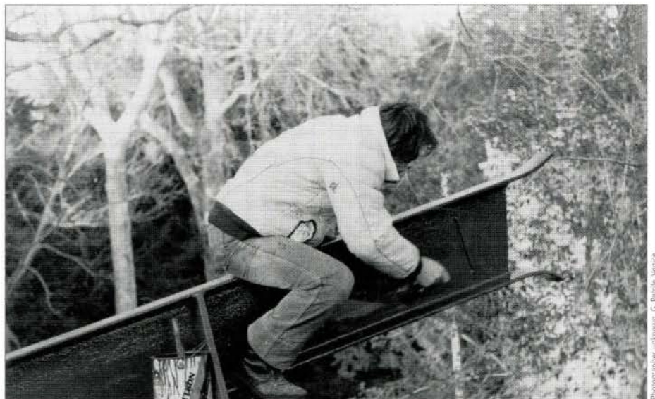
FIG. 18. EXTERIOR VIEW, DETAIL OF I-BEAM, CANADIAN PAVILION, VENICE.
