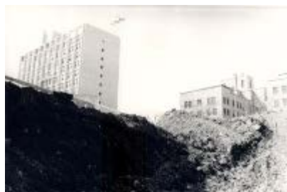
Bernard M. Cain Building - Timber Structures Laboratory - Excavation Photo - 1, 1967
