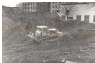
Bernard M. Cain Building - Timber Structures Laboratory - Excavation
