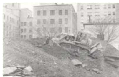
Bernard M. Cain Building - Timber Structures Laboratory - Excavation Photo - 2, 1967
