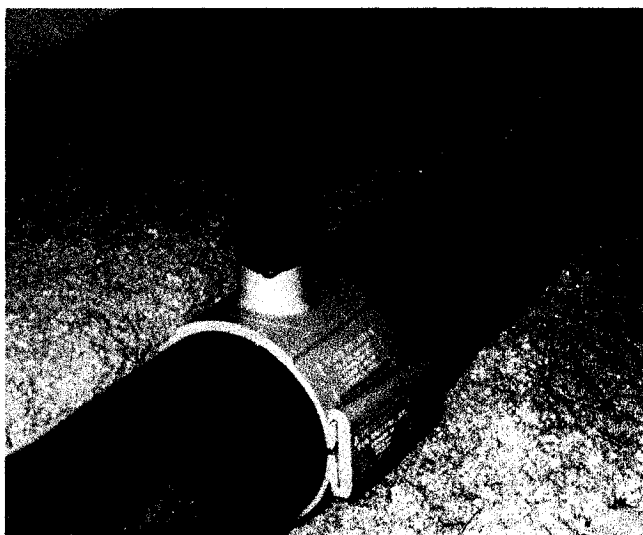
Figure 4.13: B line paddlewheel flowmeter sensor
