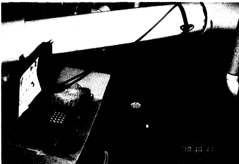
Figure 4.12: Ultrasonic flowmeter on Site D pipe
