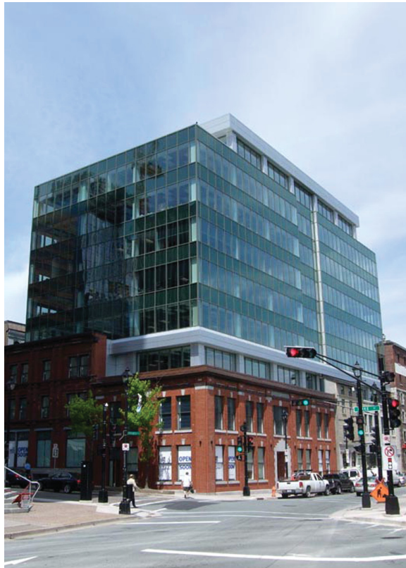
Example of Facadism in downtown Halifax. Building located at the corner of Upper Water and Duke Streets.
