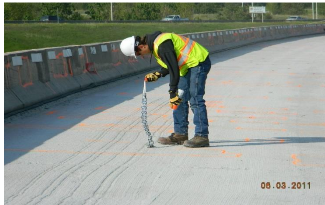
Figure 3-2: Chain dragging and delamination marking
