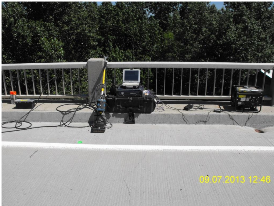
Figure 5-1: Radar equipment used for testing
