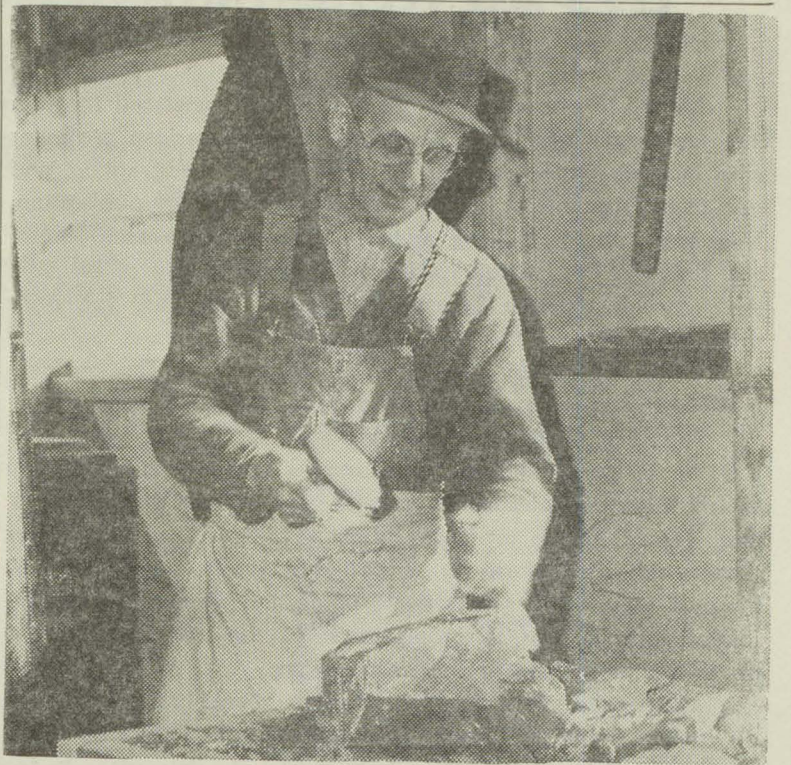
A mason is shown at work preparing stones for the new addition to Shirreff Hall. Actual construction of the new quarters will begin this spring.
