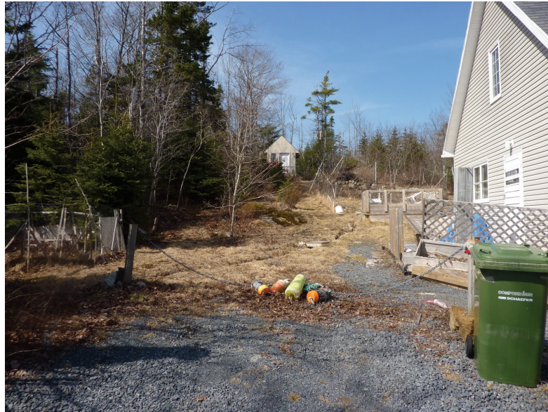
Figure C.5 Home and structures built into and alongside forested area in Spryfield, Nova Scotia, March 21 st , 2012.
