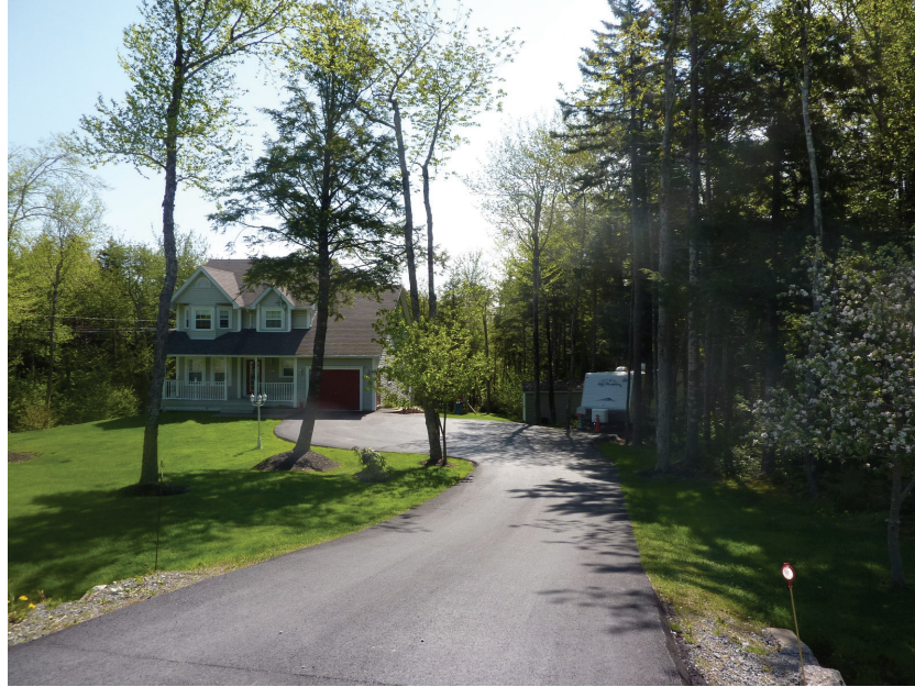
Figure C.8 Large home built into forested area in Beaver Bank, Nova Scotia, May 17 th , 2012.
