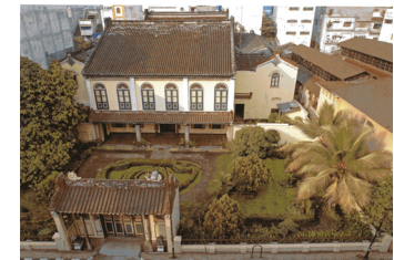
Figure 11: Tjong A Fie Mansion in Medan, Indonesia, 2010; from Ronald G. Knapp, Chinese Houses of Southeast Asia .
