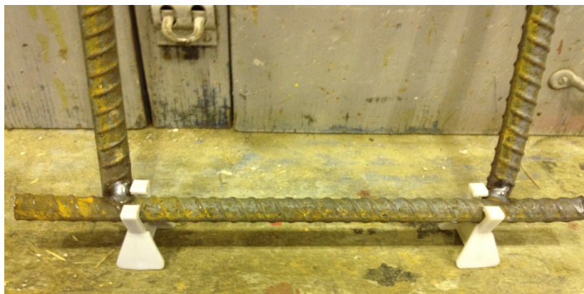
Figure 3.10 Reinforcement placed on 25 mm chair
