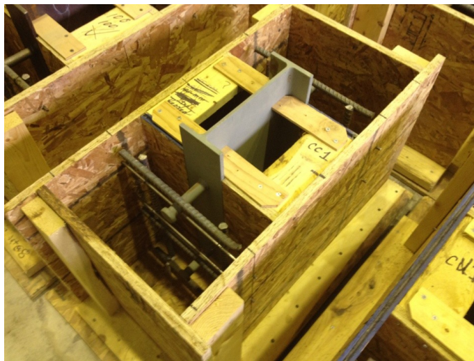
Figure 3.7 Formwork pieces
