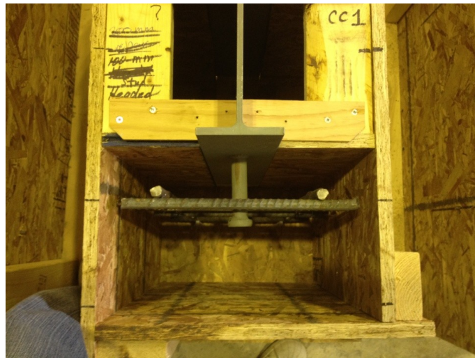
Figure 3.8 Wooden formwork for specimen S1-24-1
