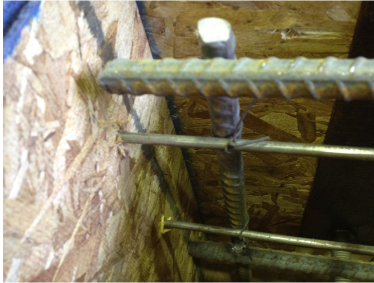
Figure 3.11 Tying of reinforcement
