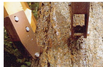
Fixed joint, knee bracket which slips onto the Garnier Limb. By Radek Kurzaj (Nelson 2004, 209).
