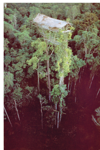
Korowai Treehouse in Papua New Guinea. Photograph by G. Steinmetz (Nelson 2004, 22).
