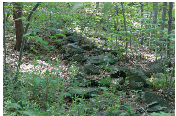
Maplewood Estate stone foundation wall.
