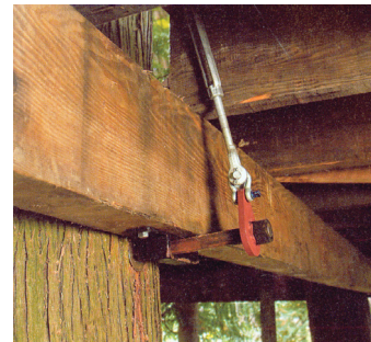
Flexible joint, looped metal bracket which slips onto the Garnier Limb. By Michael Matisse (Nelson 2004, 9).
