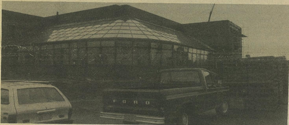
Photos of the addition to Cox Institute of Agricultural Technology.
