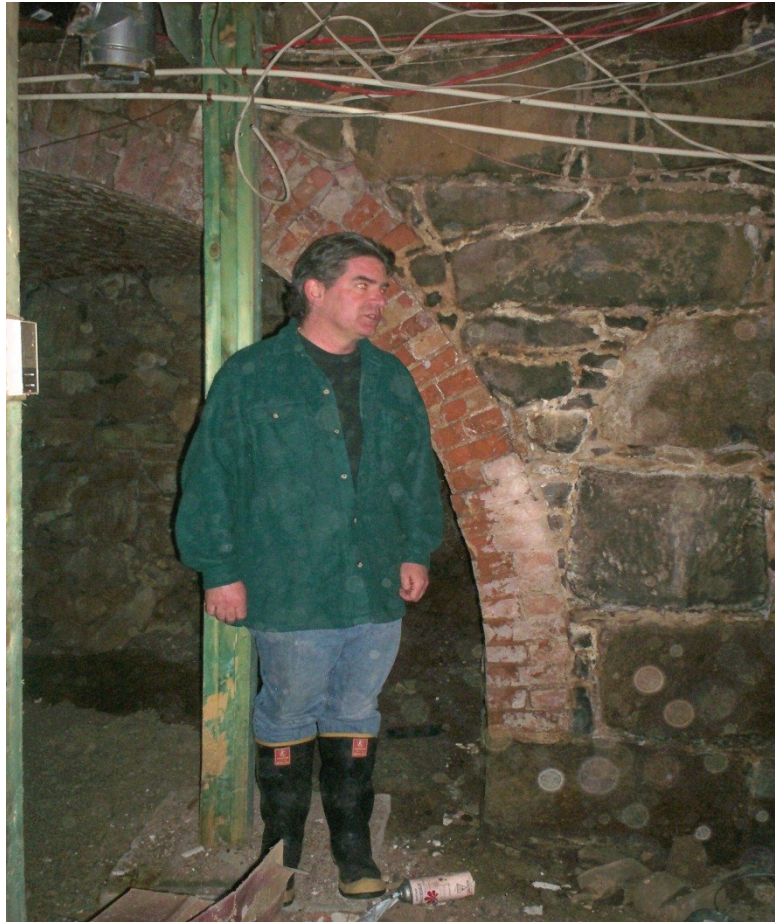
3.24 An image of the cellar feature associated with the c. 1784 home of Timothy Ruggles. The cellar lies beneath the modern home of the current landowners. The floor consists of dense, large boulders and loose soil which represents modern cellar refurbishment activities by the current landowners. (C. Cottreau-Robins, 2007)
