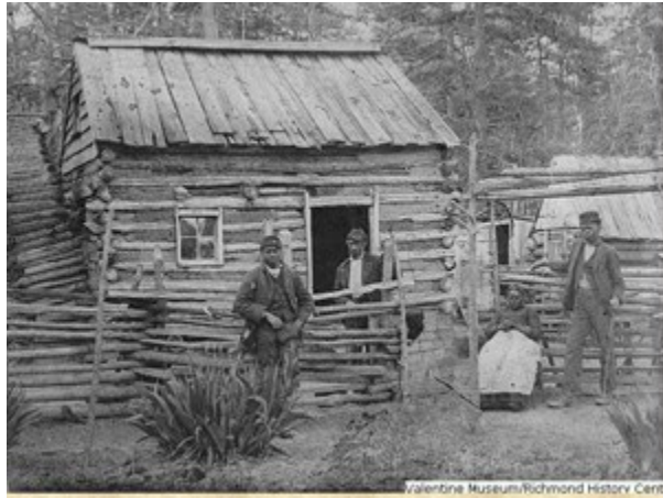
3.66 A single log house photographed near Richmond, Virginia in the late nineteenth century. Except for the glass window, it is representative of a typical log cabin described by former slaves. Something similar may have been at the cabin site in the Elliott field. Evidence of an external chimney was not recorded and it is likely that clapboard covered the exterior. A dry laid stone foundation was recorded whereas in Virginia many slave quarters were earthfast construction especially in the eighteenth century. 342
