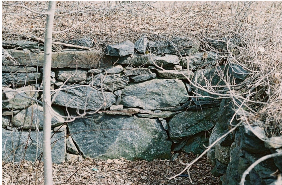
4.12 Possible nineteenth-century foundation on the Ruggles property in the treed area to the north east of the stone erratic. (C. Cottreau-Robins, 2008)
