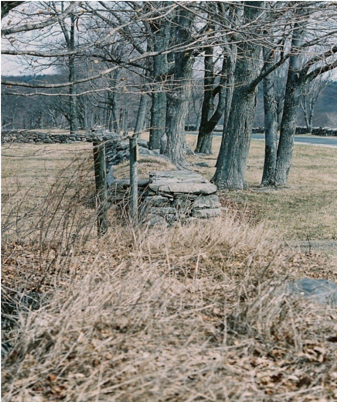
4.5 Handmade, dry-laid stone walls around the Ruggles Hardwick lands. Such walls are often associated with the eighteenth century but whether these were constructed during Ruggles' occupation is unknown. (C. Cottreau-Robins, 2008)
