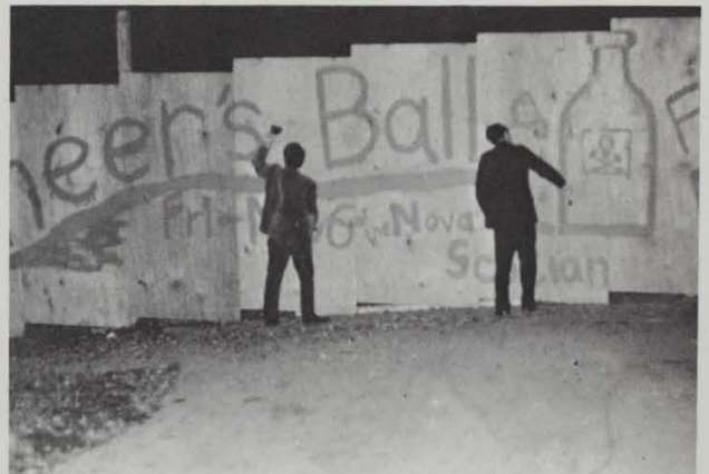
Some Engineering students make a contribution at the construction site.
