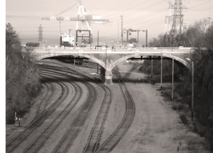
Rail cut at widest point, looking east toward Halifax Harbour. Ocean Terminal in background.
