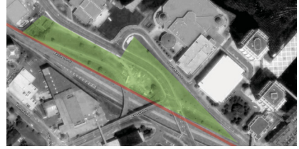
Cogswell Interchange. Google Earth image with overlay.
