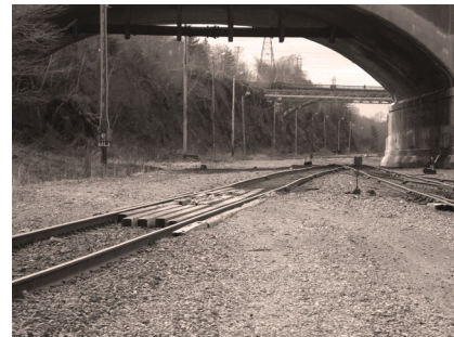
Railway looking west into the cut.
