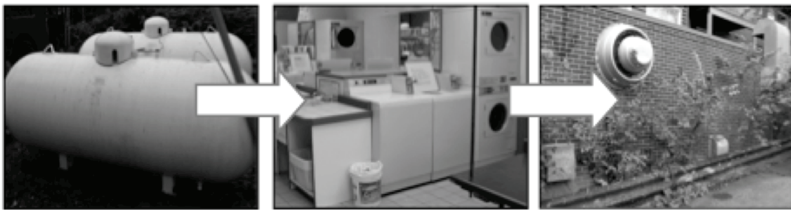
Figure 5. Commercial laundromat energy flow from propane to hot air exhaust
