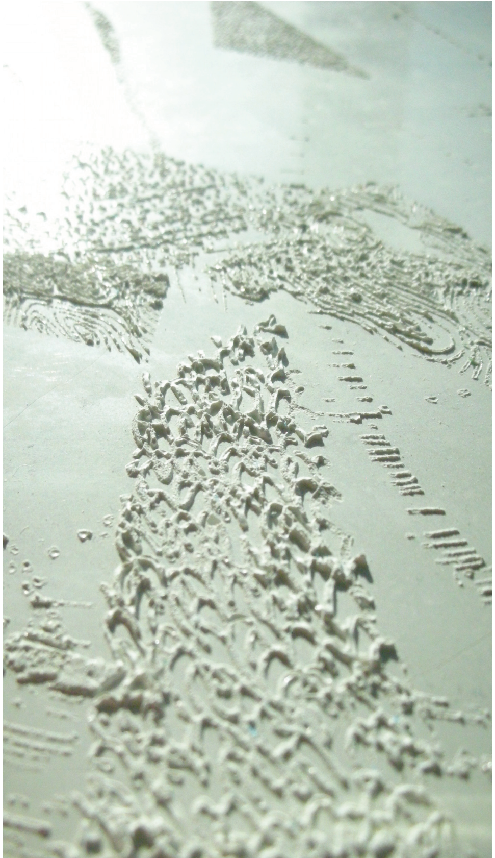
Detail of the concrete relief panel. The hand easily reads the defined lines.
